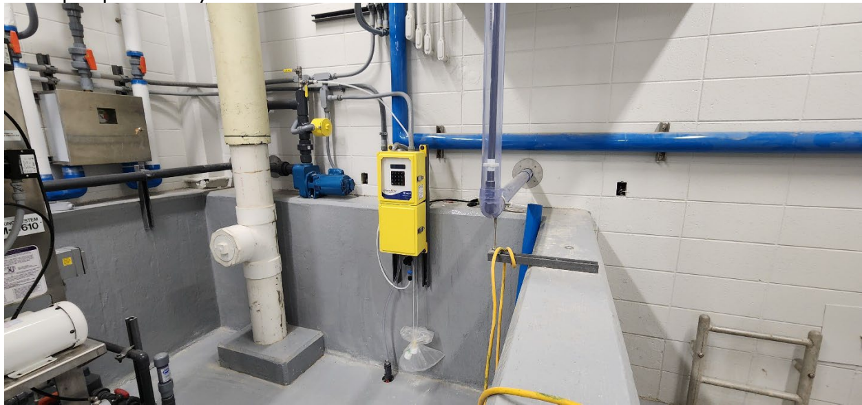
Containment area sump level sensor installed in Chemical Storage Room
