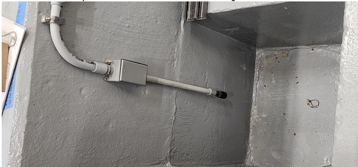
Containment area sump level sensor installed in Chemical Storage Room
