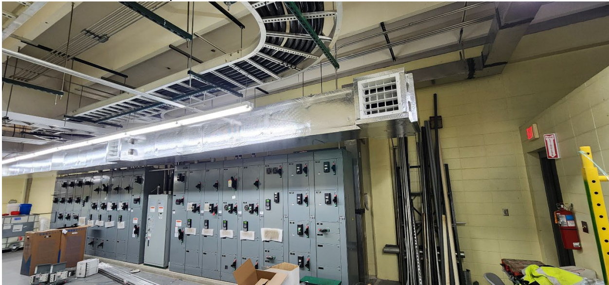
HVAC duct work insulation placed in mezzanine electrical room
