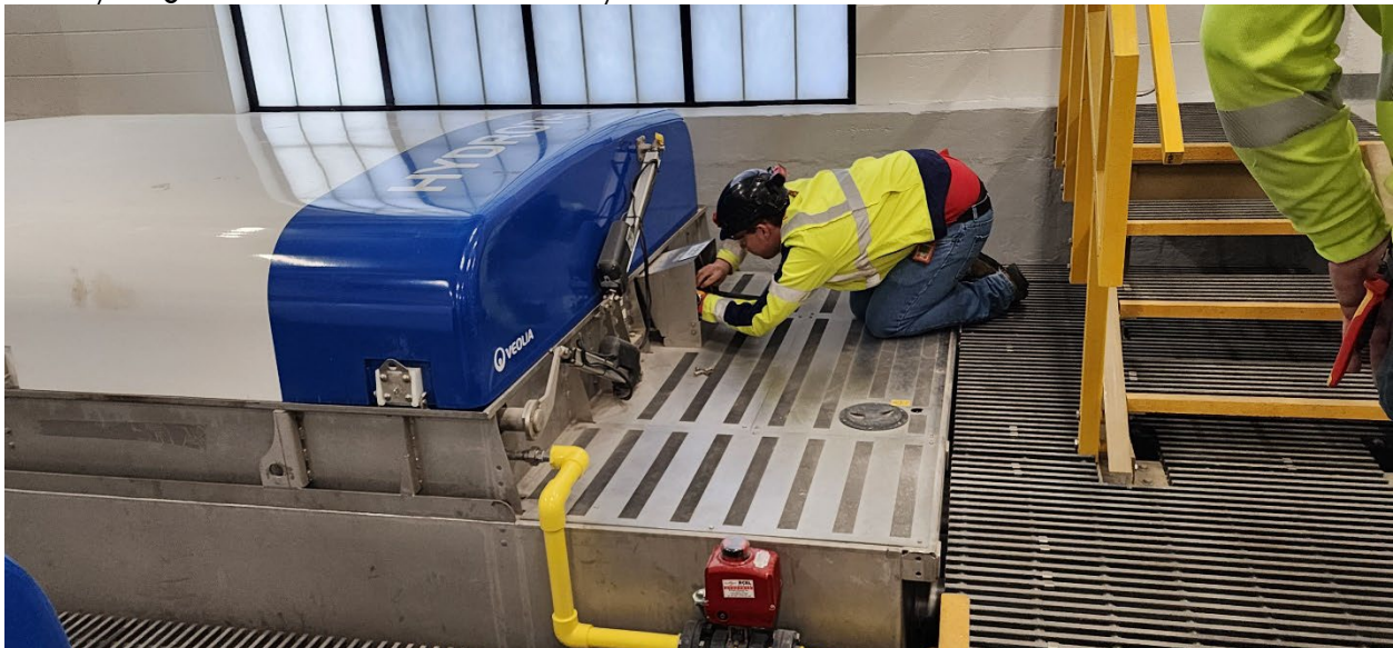
Veolia/Kruger onsite for Mechanical and I/O Checkout of Disc Filters
