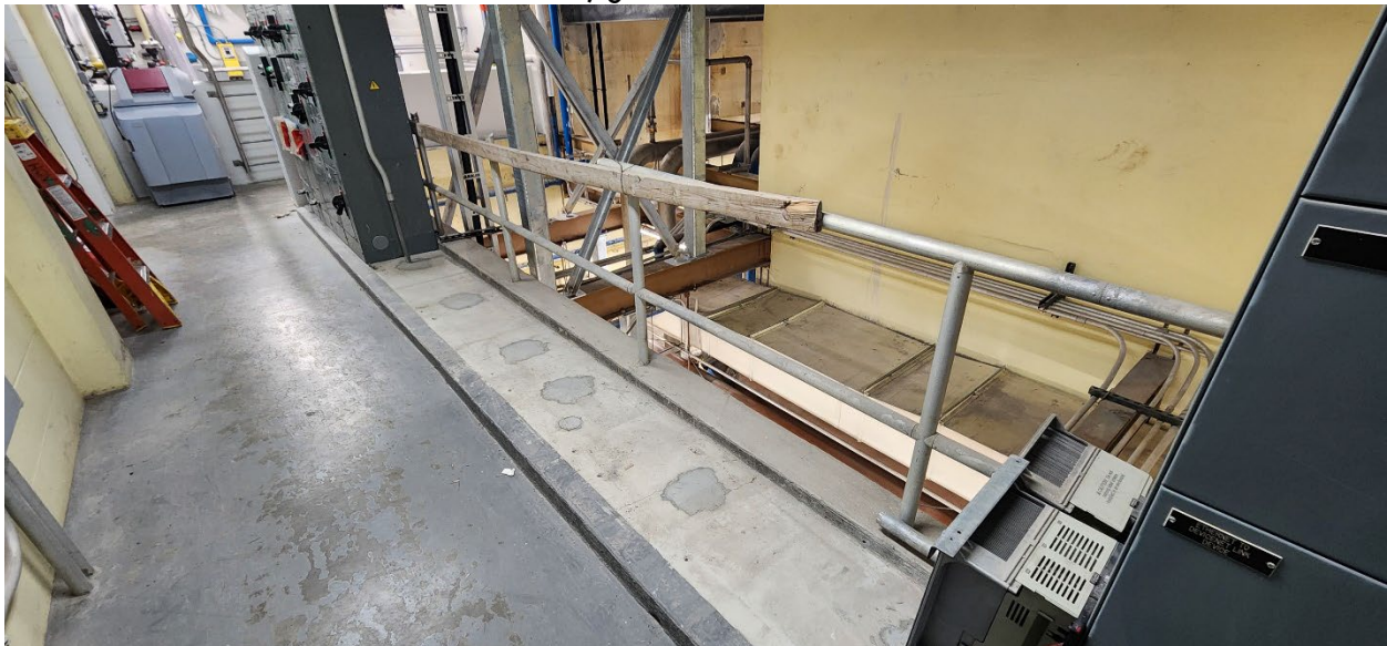
Area cleaned out between electrical units, guard rail to be reinstalled
