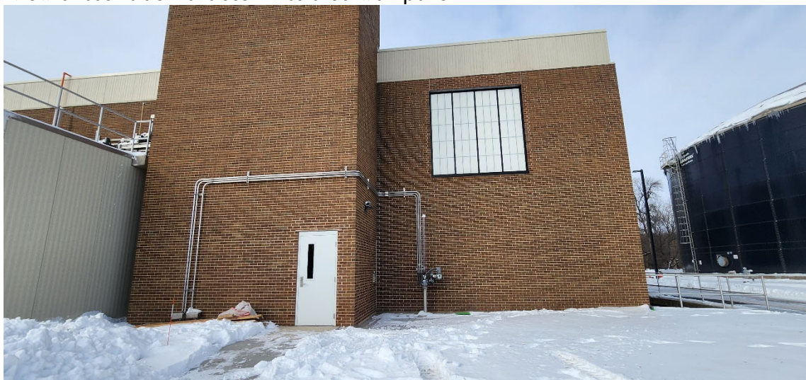
Exterior view of southside translucent insulated wall panel
