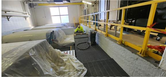
New FRP grating steps and rail to doorway to access top of new Filter Splitter Box.
