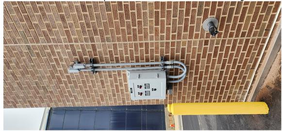
South Str 60 mandoor with new conduit runs for CCT Transfer Box gate and Chlorine Contact Tank
