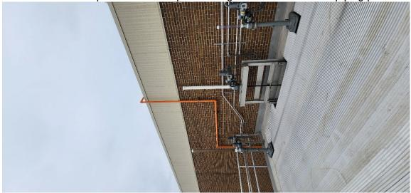
Natural gas piping painted on roof and exterior of Structure 60 and Chemical Storage, Safety Orange
