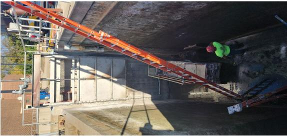
New guard rail and grating installed by the new gate for the Chlorine Contract Tank
