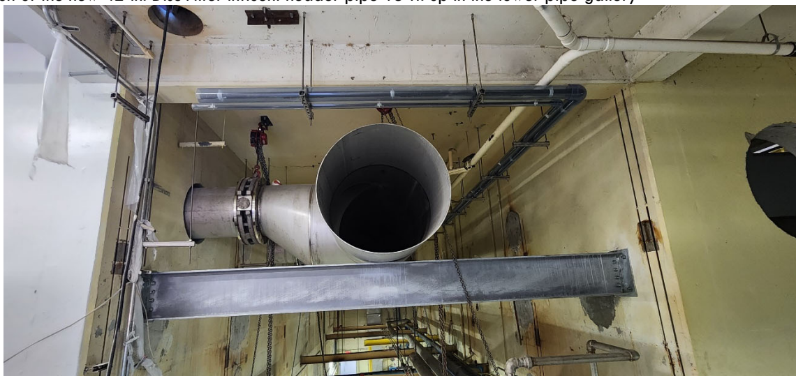
Installation of the new 42-in. Disc Filter Influent header pipe 15 ft. up in the lower pipe gallery
