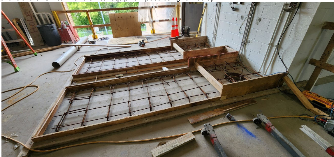
Future Muriatic and SHC Disc Filter chemical equipment pads being formed up
