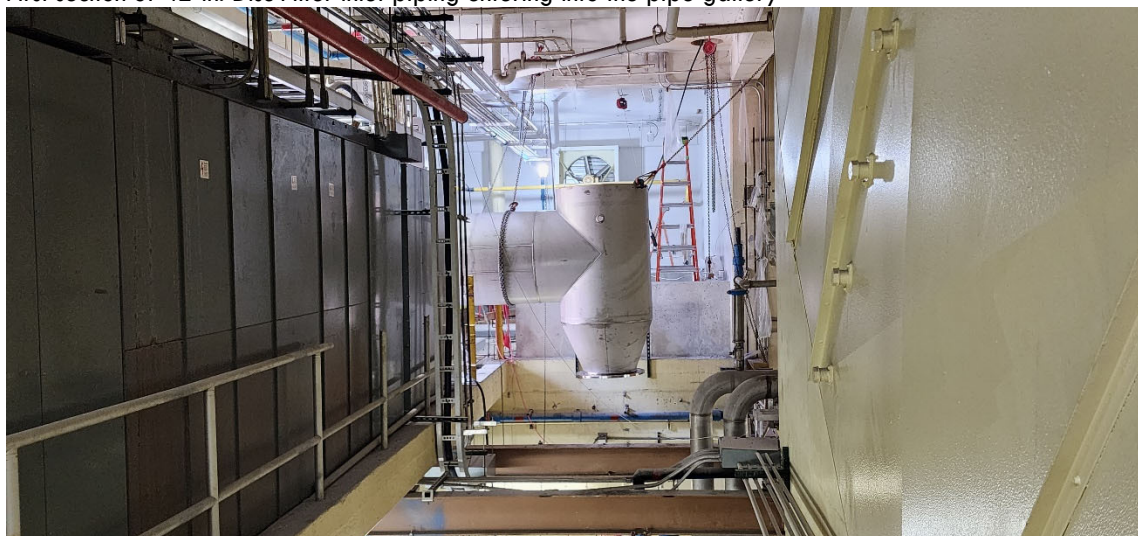
First section of 42-in. Disc Filter inlet piping entering into the pipe gallery
