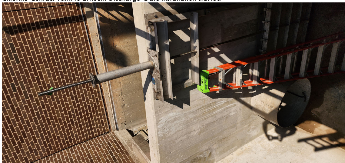
Chlorine Contact Tank to Effluent Discharge Gate installation started
