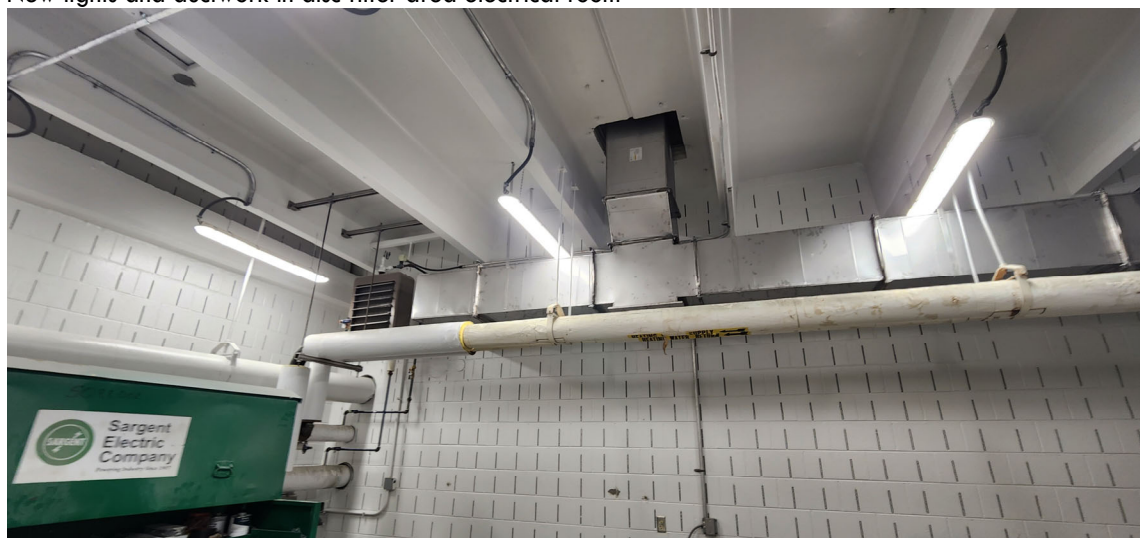
New lights and ductwork in disc filter area electrical room
