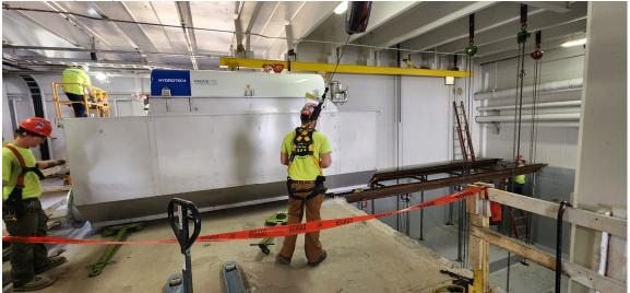
Disc Filter #1, in and Disc Filter #2 next in line to get set
