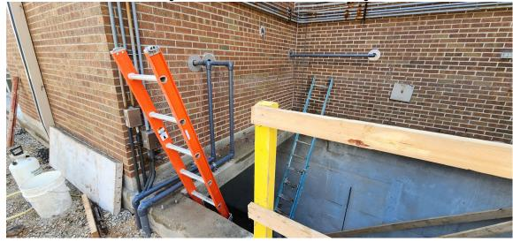
CD Smith poured the discharge baffle wall in the chlorine contact tank, with AW placed 42-in. Disc Filter Effluent pipe sleeve
