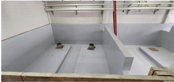
New drain and backwash waste lines entering into back wash waste well
