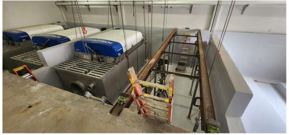
Rapid mix and coagulation basins, wall coating completed by Omni
