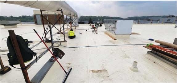
Pipe bollards getting set and placed to be poured in around Chemical Storage Room, mandoor stoops poured
