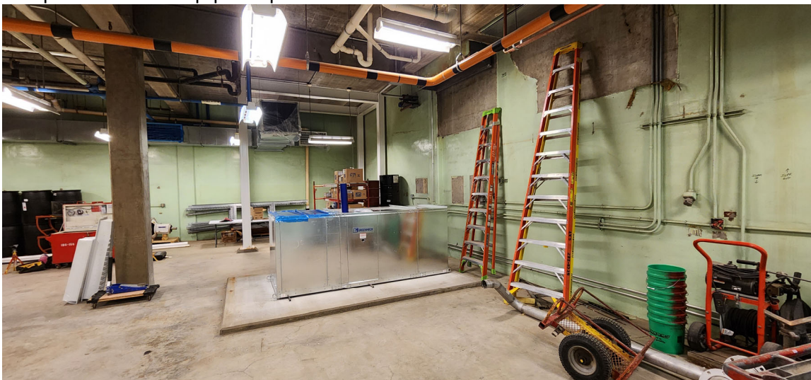
New Make Up Air unit set on equipment pad in lower lever Boiler Room
