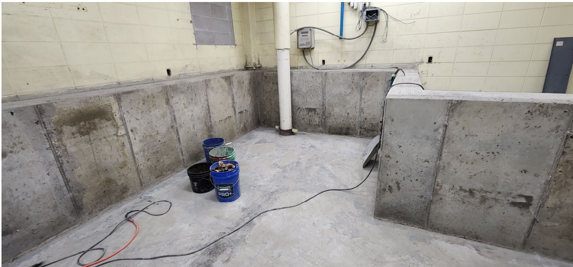
New containment walls for chemical feed room
