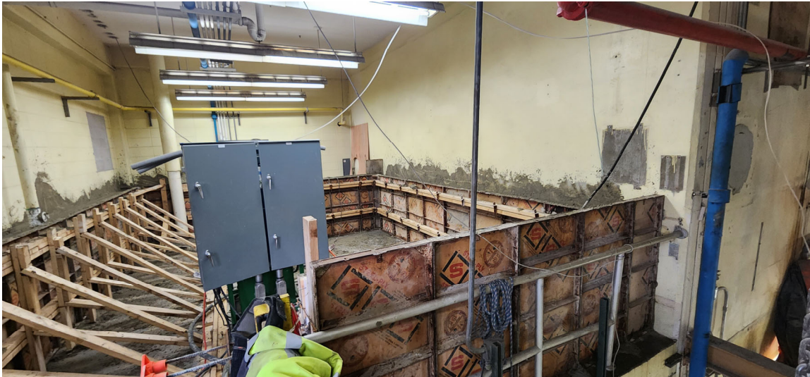
Formwork set for chemical feed room containment walls in Str 60
