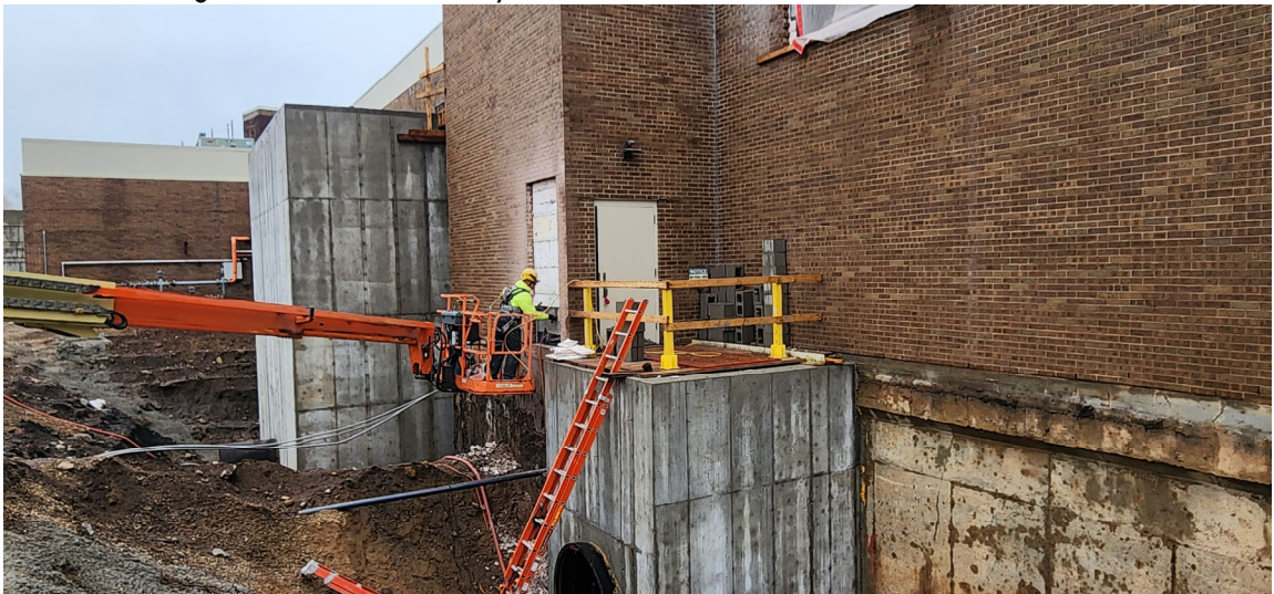
CD Smith Masons cutting in new south door way near CCT Transfer Box
