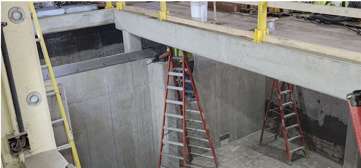
Installation of Flocculation basin weir
