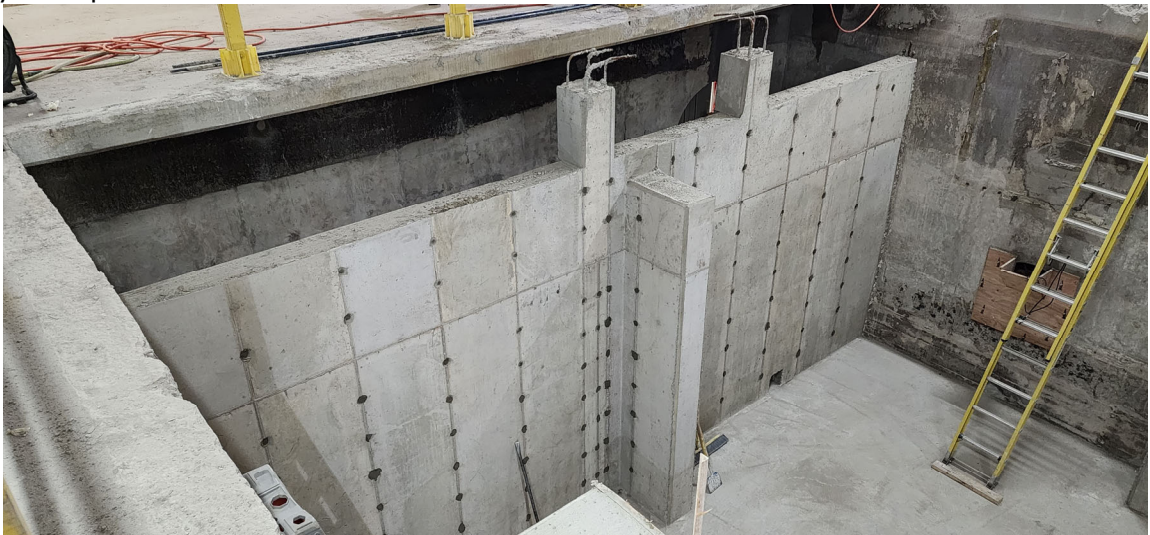
Flocculation basin north weir wall concrete complete, waiting for weir plate, coating, basin walkway to be placed
