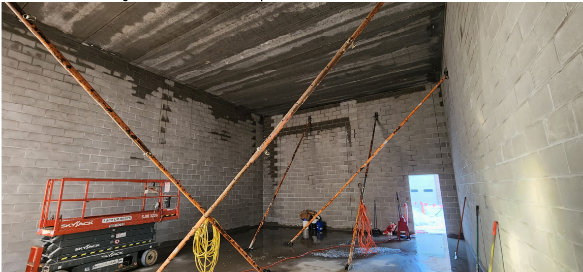
Interior of the chemical storage room with new roof planks set
