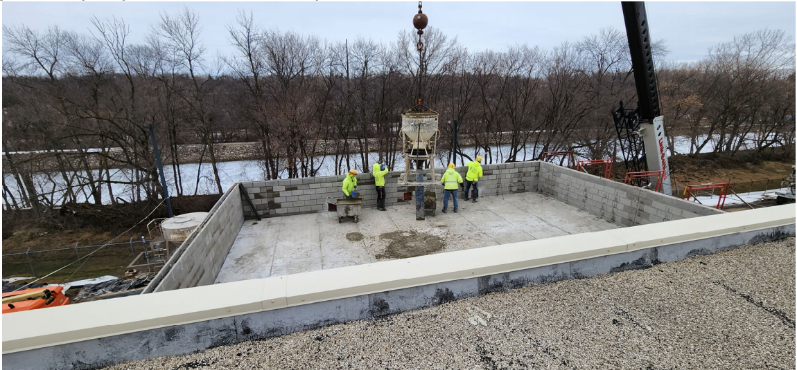
Flocculation basin north weir wall concrete complete, waiting for weir plate, coating, basin walkway to be placed
