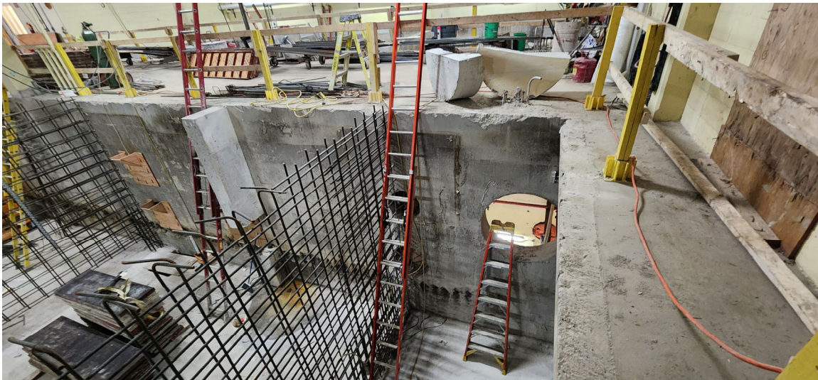
New pipe core completed for 42" filtration pipe in filtration basin prior to entering the Filter Splitter Box
