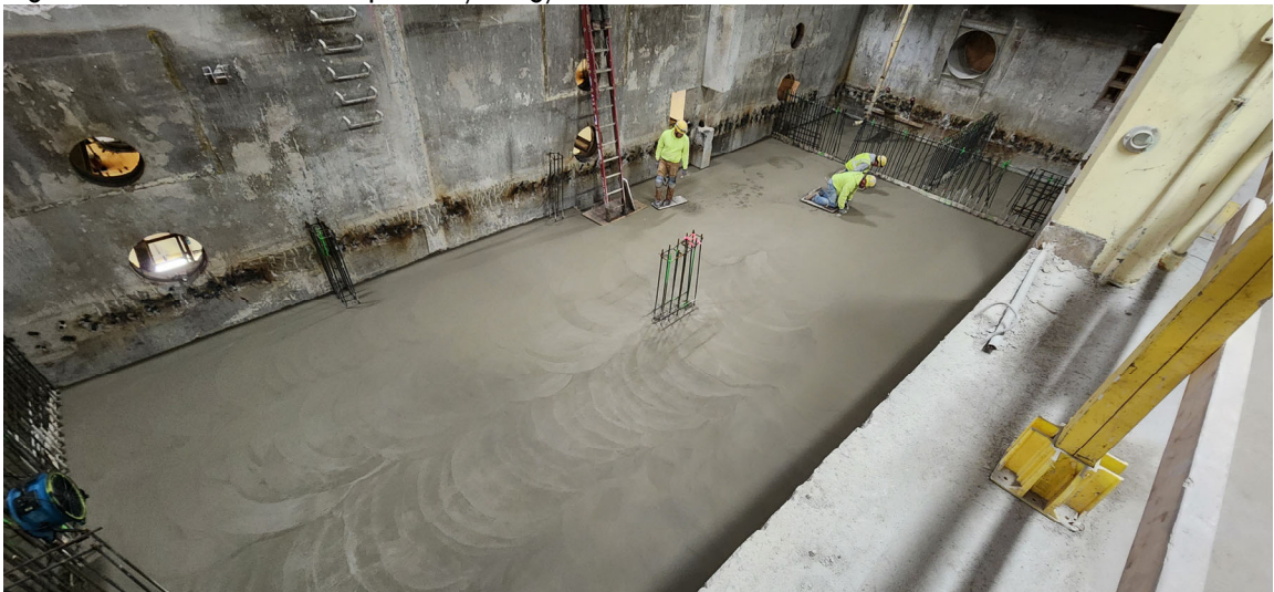
Completing the floor finish for the rapid mix/coag/floc floor slab
