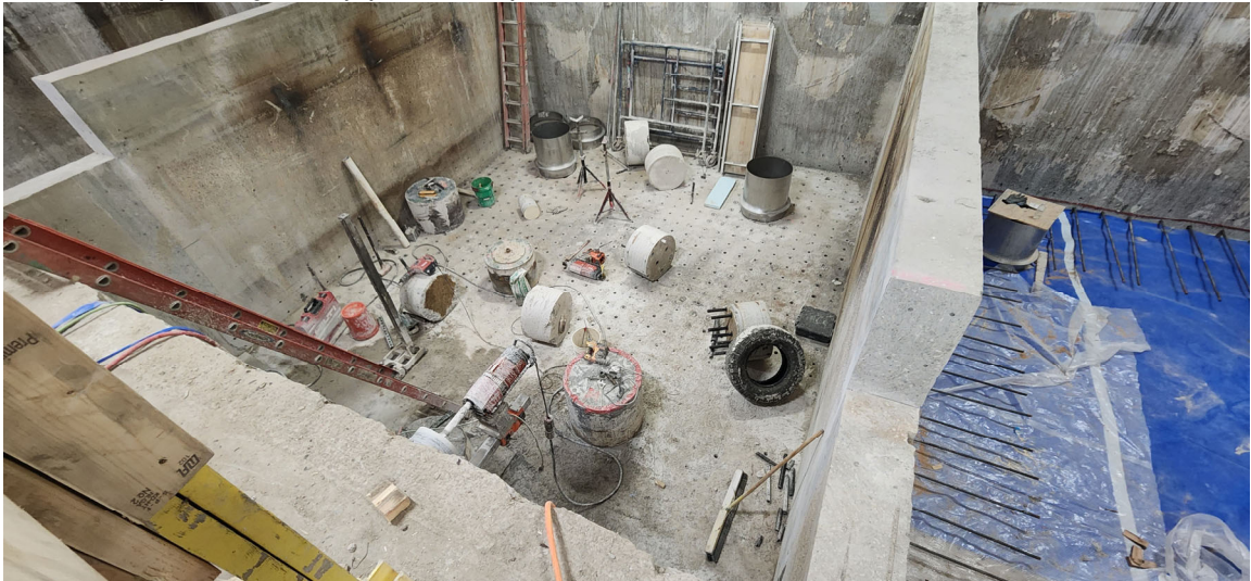
North Disc Filter bay floor rebar and pipe sleeves placed
