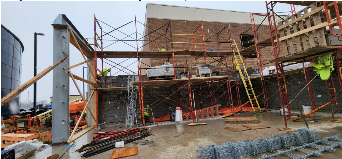
Mason starting on CMU wall for Chemical Storage room and placement of OHD frame on east side
