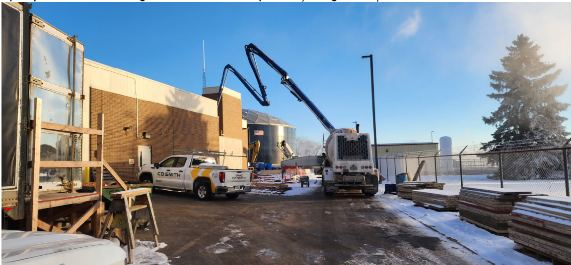
Concrete pumper truck delivering concrete to new rapid mix/coagulation/flocculation floor slab
