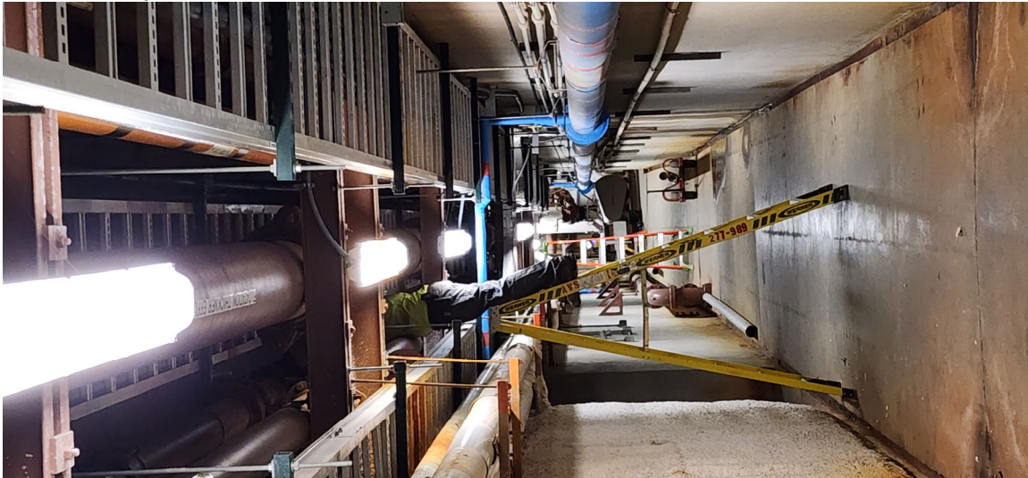
New pipe core completed for 42" filtration pipe in filtration basin prior to entering the Filter Splitter Box
