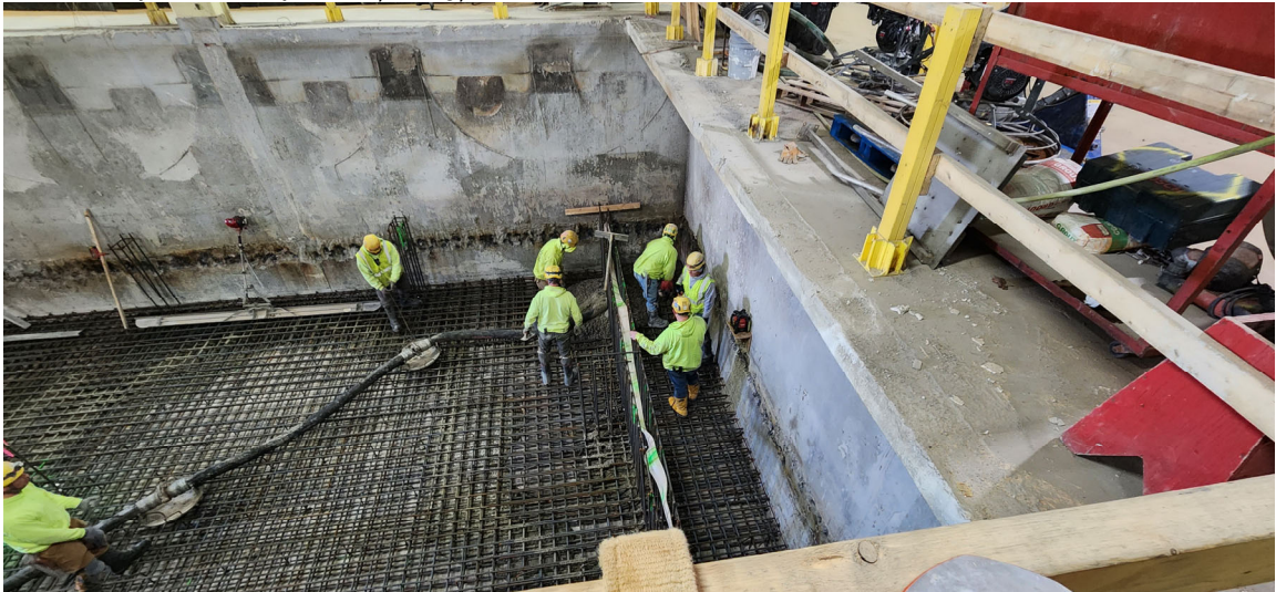
Completing the floor finish for the rapid mix/coag/floc floor slab
