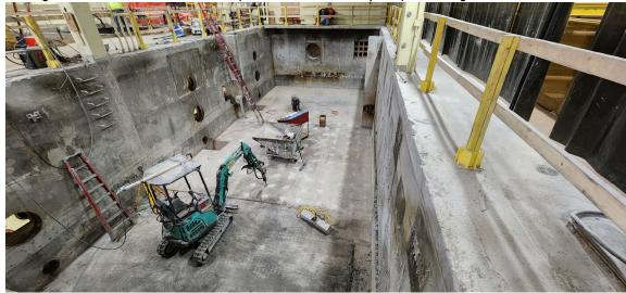
54" pipe sleeves for new CCT Transfer Box placed on base slab
