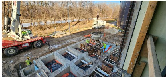
Rm 122 grade beam and foundation insulation being placed
