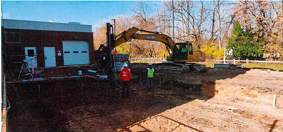
Terra installing first grouted micropile for new Str 122 Filter Chemical Storage
