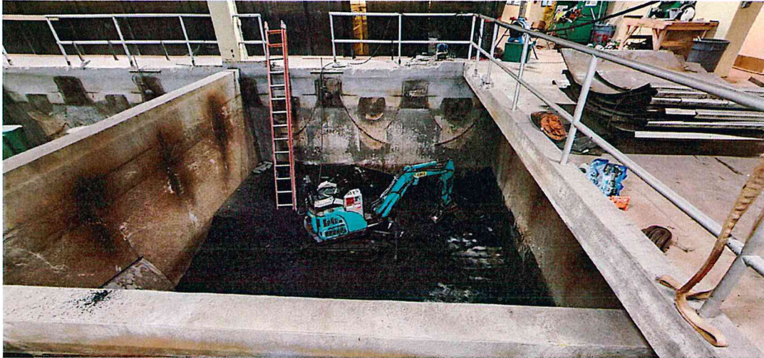
Anthracite being removed from old filters, prior to concrete demolition in Str 60.
