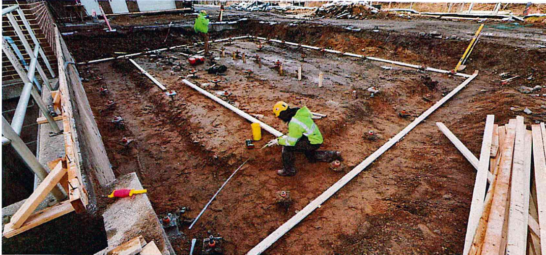
Grouted micropiles complete for Str 122 Filter Chemical Storage grade beams, CD Smith starting formwork
