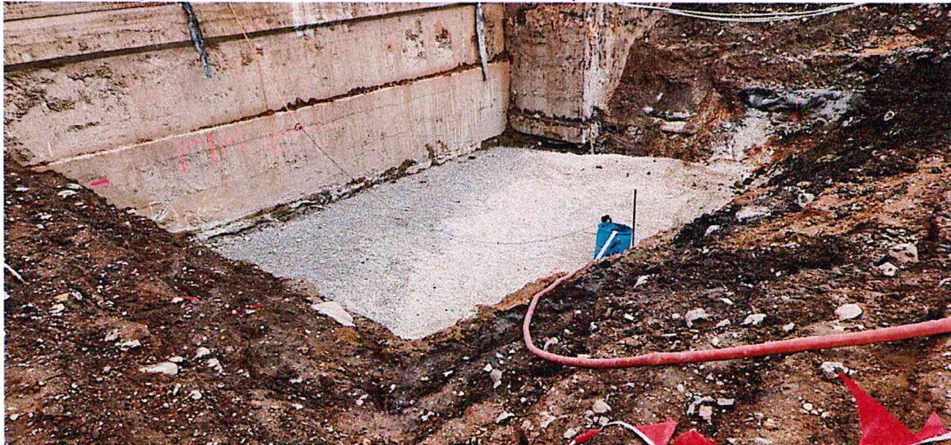
Foundation base ready for rebar and concrete for Str 123 Filter Splitter Box
