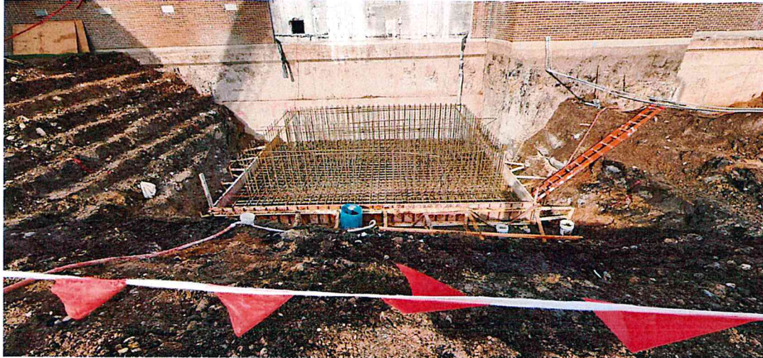
Grouted micropiles complete for Str 122 Filter Chemical Storage grade beams, CD Smith starting formwork
